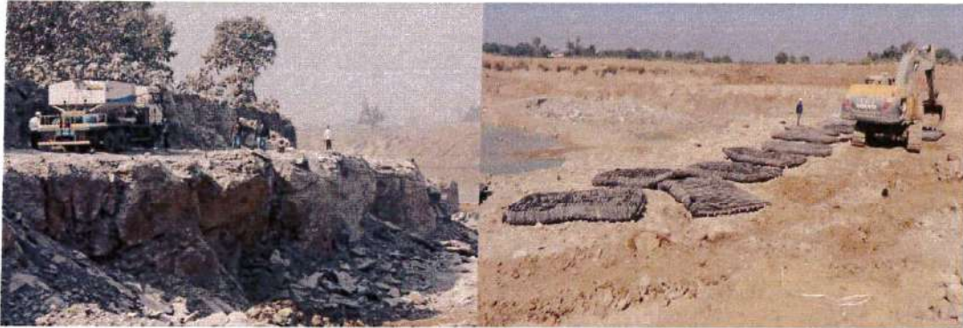
Photograph 2. The charging of the 15 no. RPL bench and use of blasting mate at 7050 RIL blast face to prevent flyrock.
