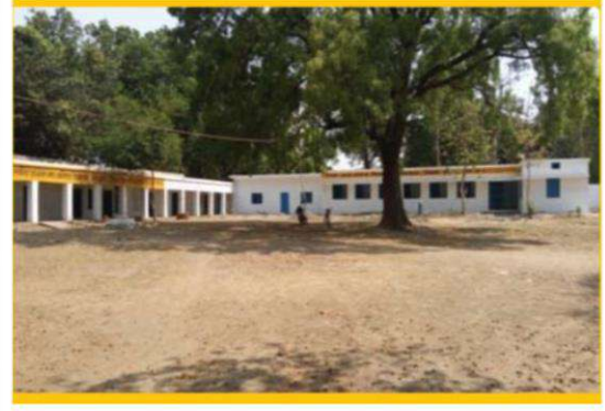
Renovation of Hr. Sec. School at Sijhata
